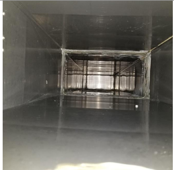
After Duct Cleaned
