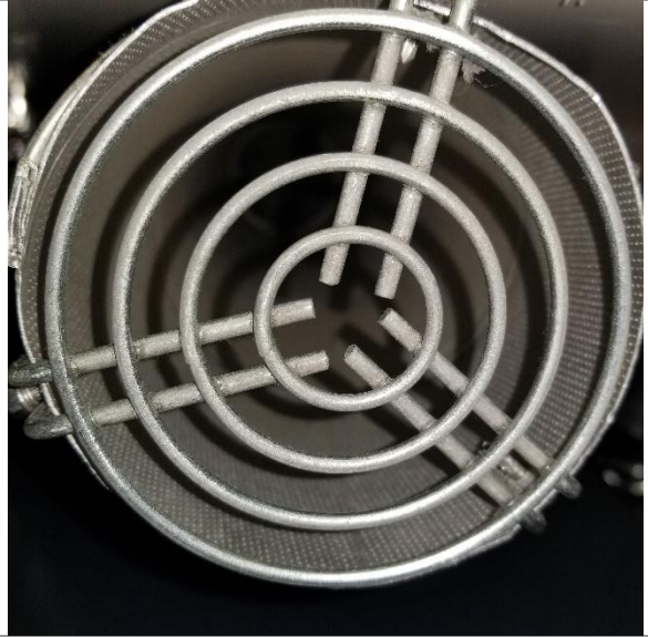
After Register Cleaned
