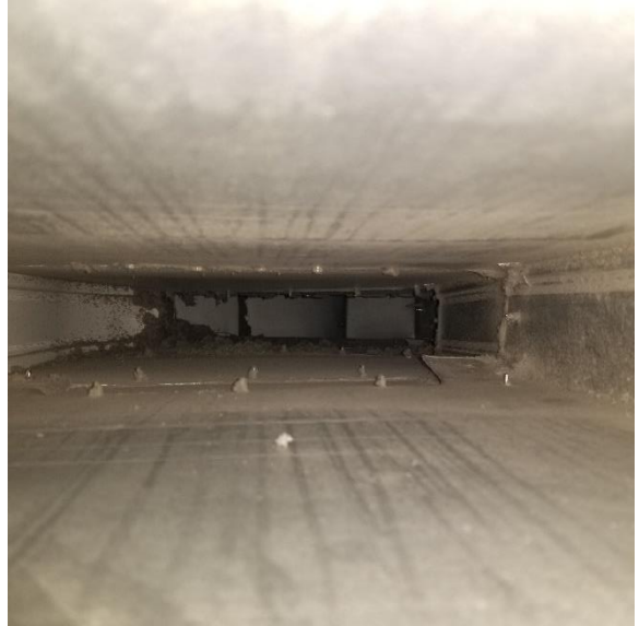
After Duct Cleaned
