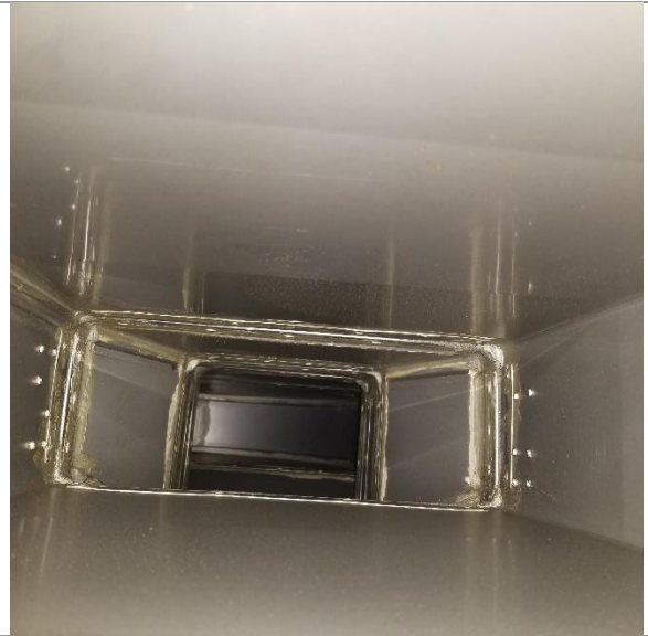
After Duct Cleaned
