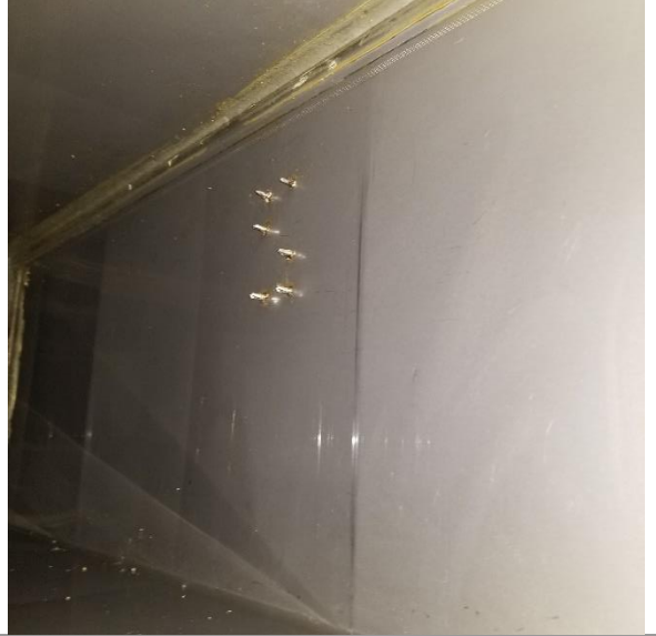
After Duct Cleaned
