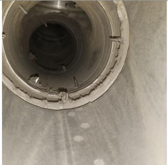
After Duct Cleaned
