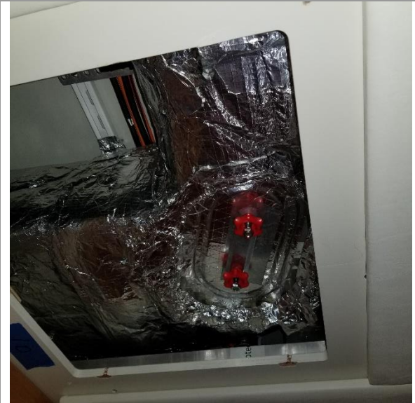
AFTER Access Sealed
