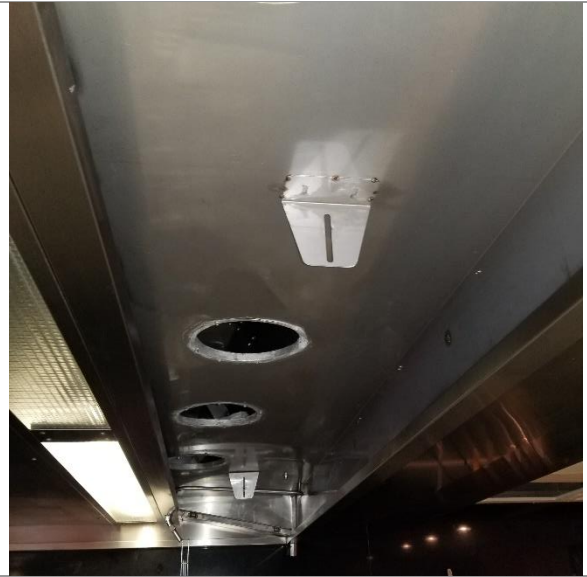
After Area Cleaned
