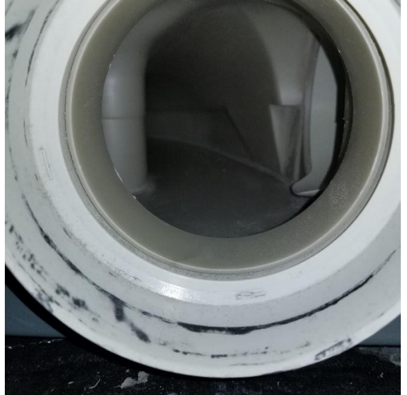
After Area HEPA Cleaned
