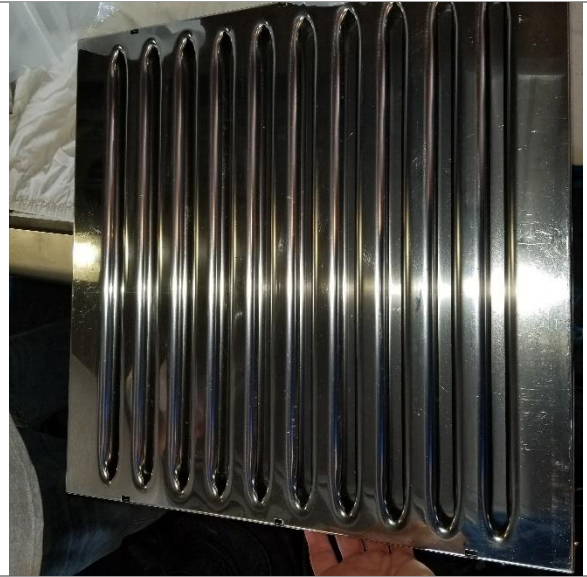
After Baffles Cleaned
