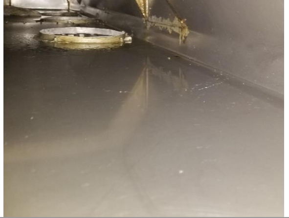
After Duct Clean
