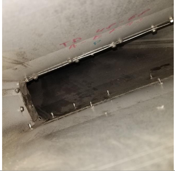
AFTER Duct Cleaned
