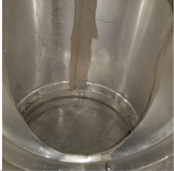
AFTER HEPA Vacuumed Cleaned
