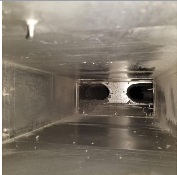
After Duct Cleaned
