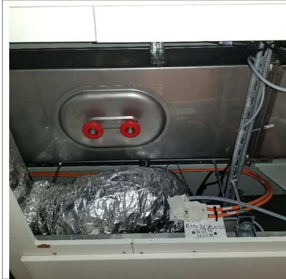
Before Exhaust System Access Sealed
