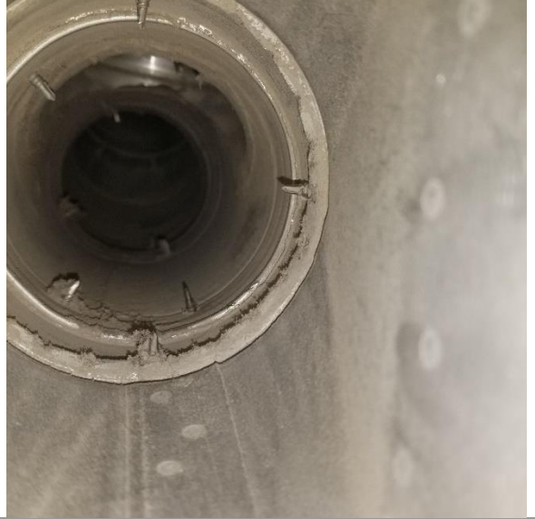
After Duct Cleaned
