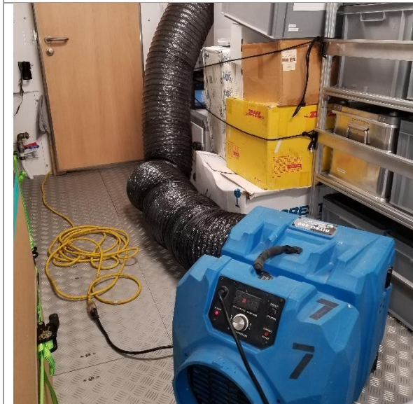
HEPA Negative Air Implemented
