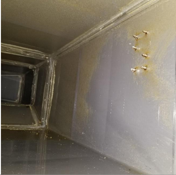
BEFORE Walls Partially Cleaned
