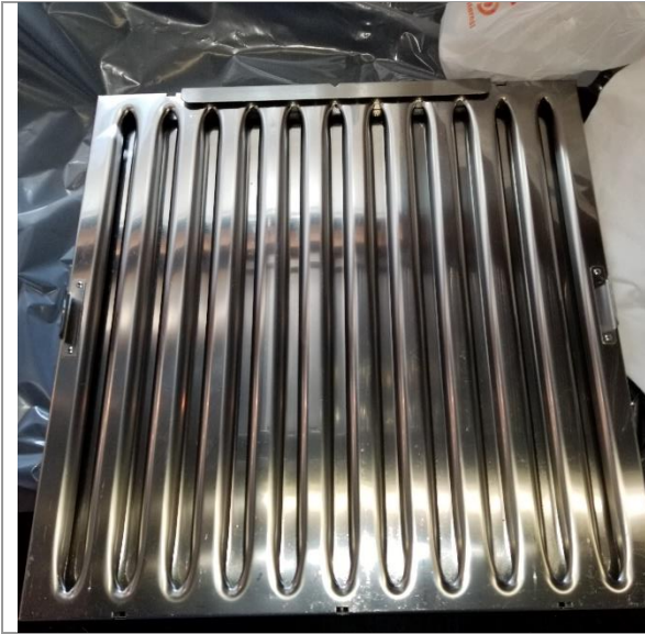
Before Baffle Filters with Slight Grease
