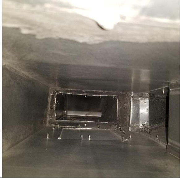
After Duct Cleaned
