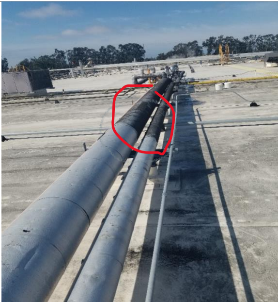
In Cleaning Process All pipes cleaned the same manner with same results (Note Color Difference)
