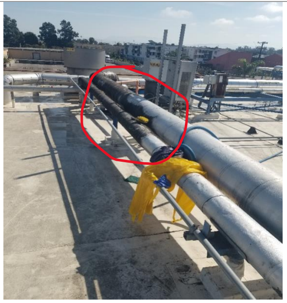
In Cleaning Process All pipes cleaned the same manner with same results (Note Color Difference)
