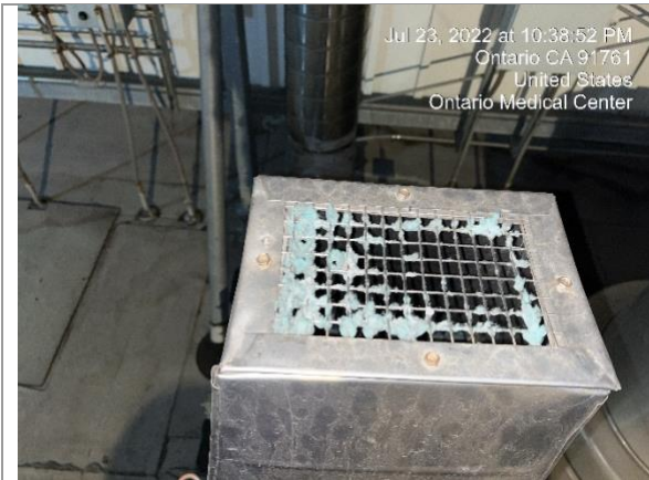
Before Exhaust Port on Rooftop
