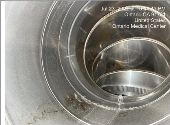
Before Duct Work
