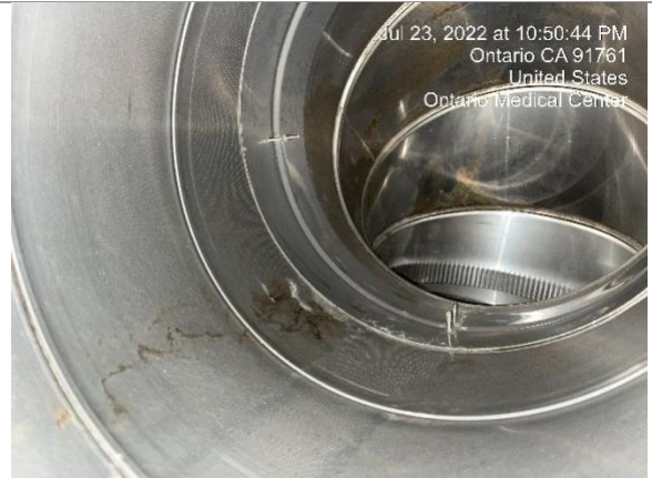
After Duct Work
