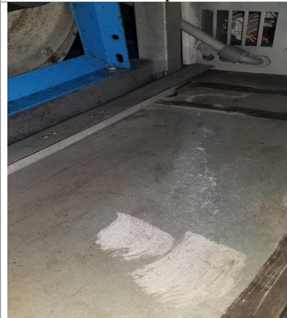
Before Coil Area
