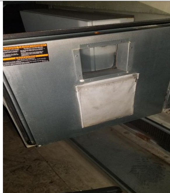
After Interior of Access Doors
