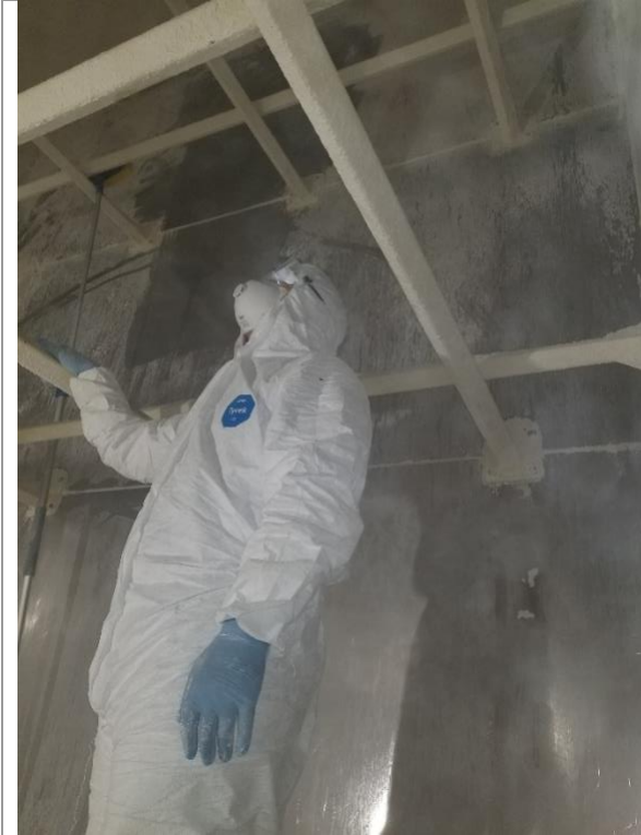
Team members wearing proper PPE
