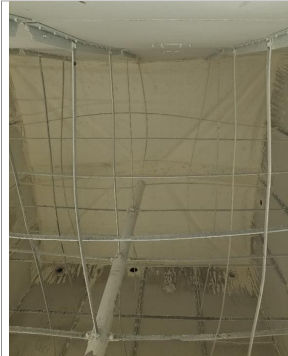
Before Ceiling and bars
