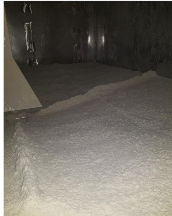
Before Interior floor
