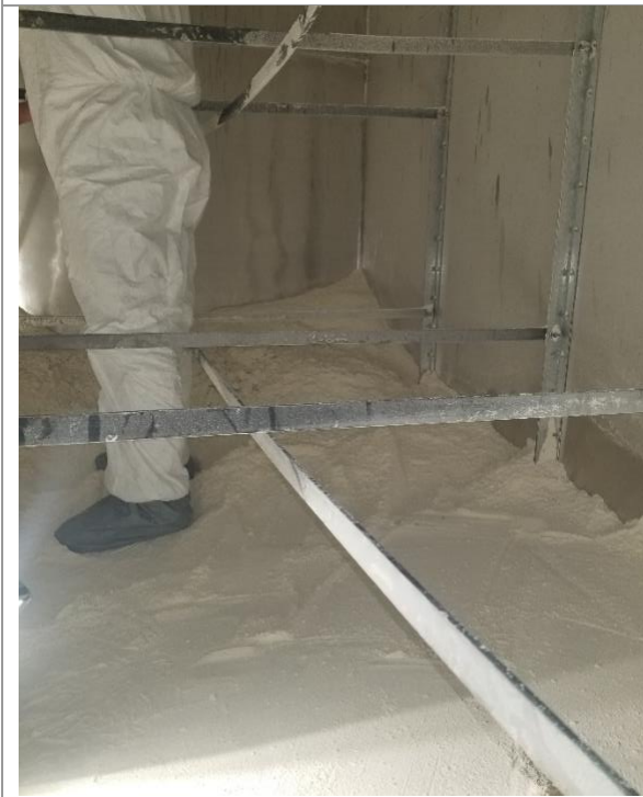
Before Interior floor
