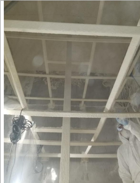
Before Ceiling and bars
