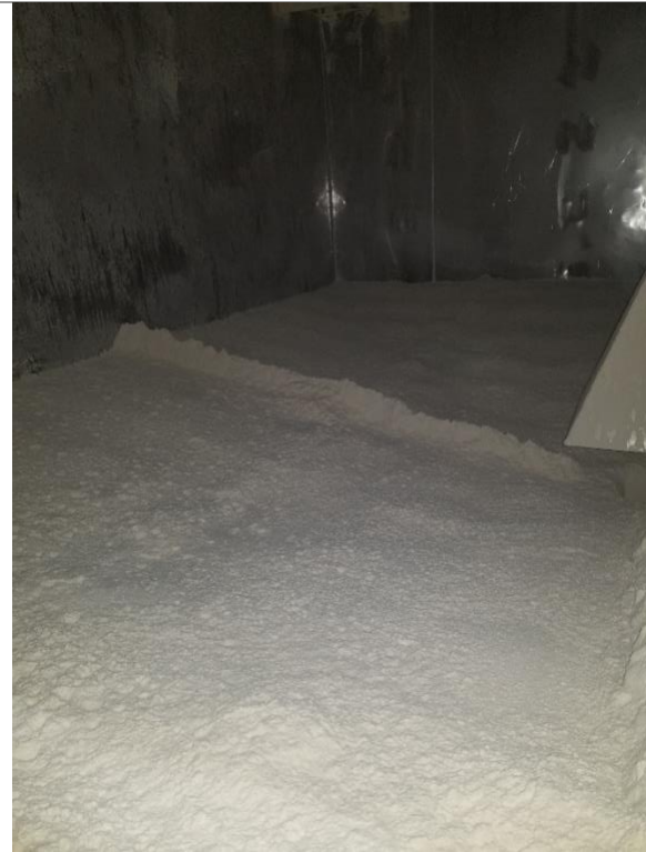
Before Interior floor
