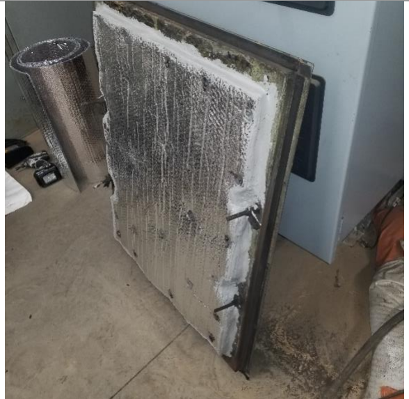
---After--- AstroShield repair to resolve debris issue from doors
