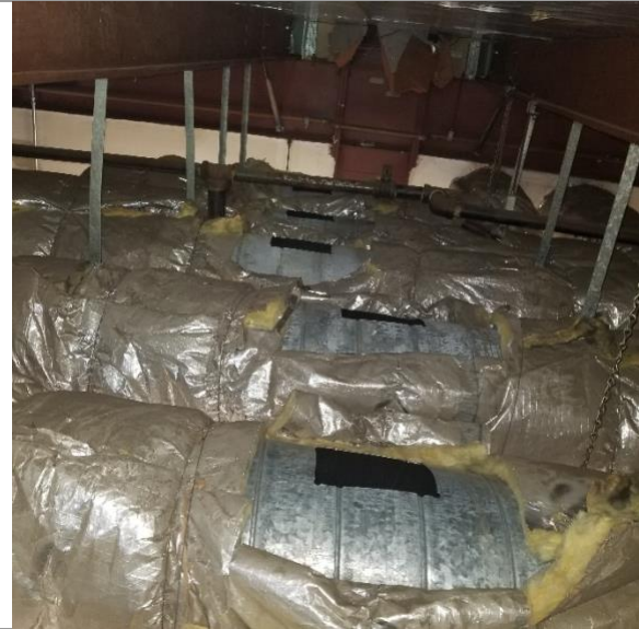
Access created to inspect and clean
