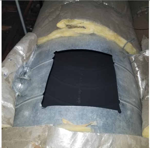
Access created to inspect and clean
