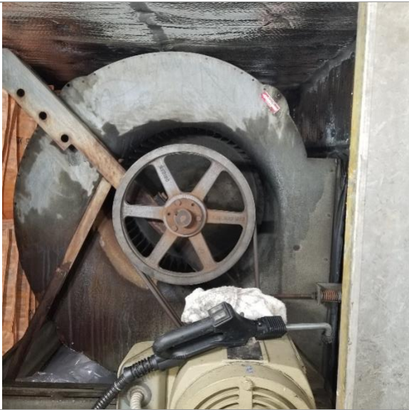
Steam cleaning in progress
