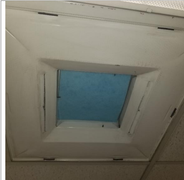
--After-- cleaning filter media added
