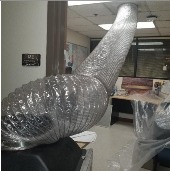
-Methodology- cleaning ducts, HEPA negative air
