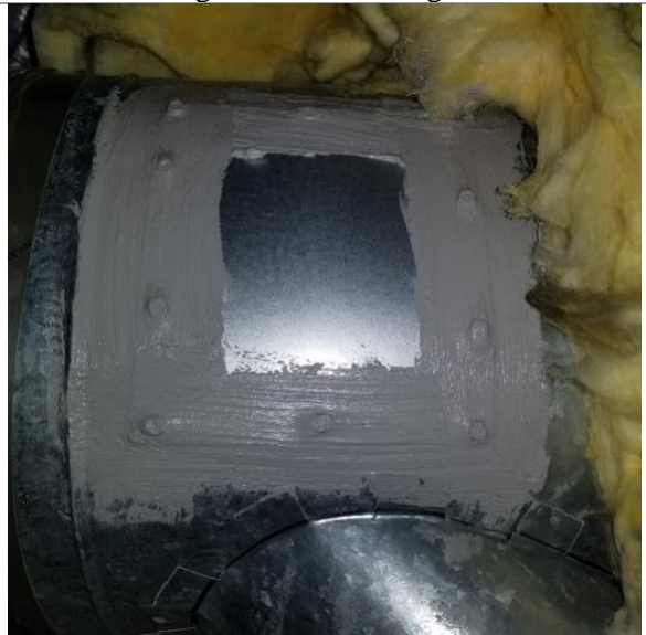
---After--- Sealed (Typical for all access points)
