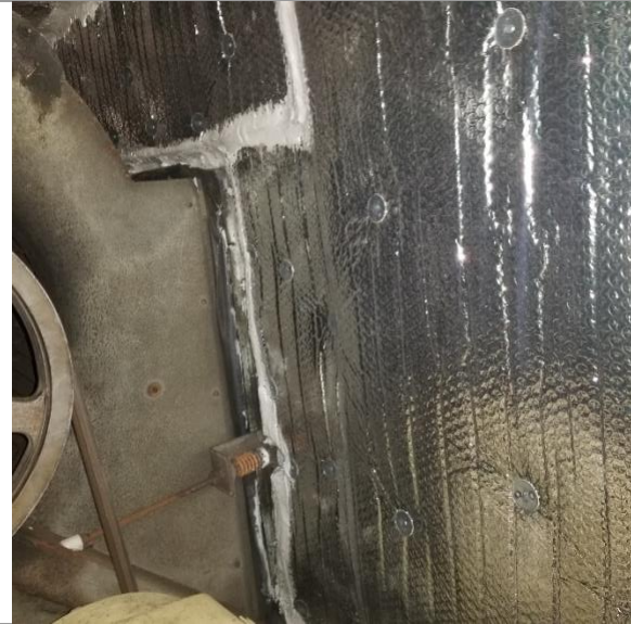
---After--- AstroShield repair to resolve debris issue from unit
