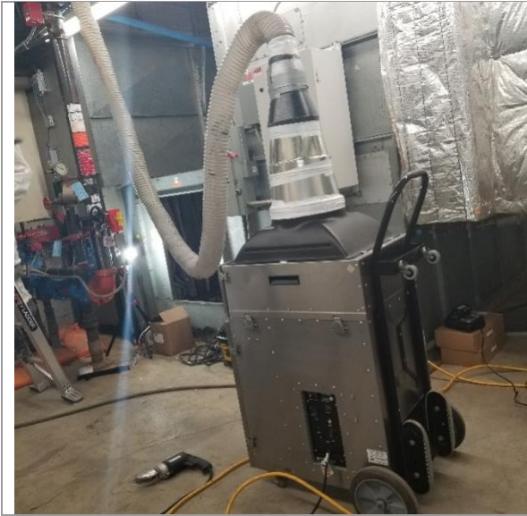
HEPA negative air used to clean mechanical area
