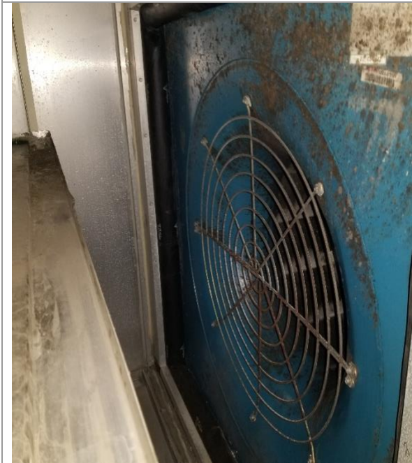
--Before-- Fan with debris and organic growth
