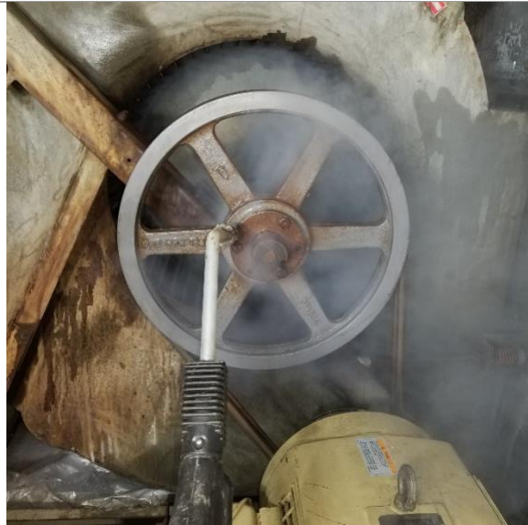
Unit steamed cleaned. Process also eliminates organic growth
