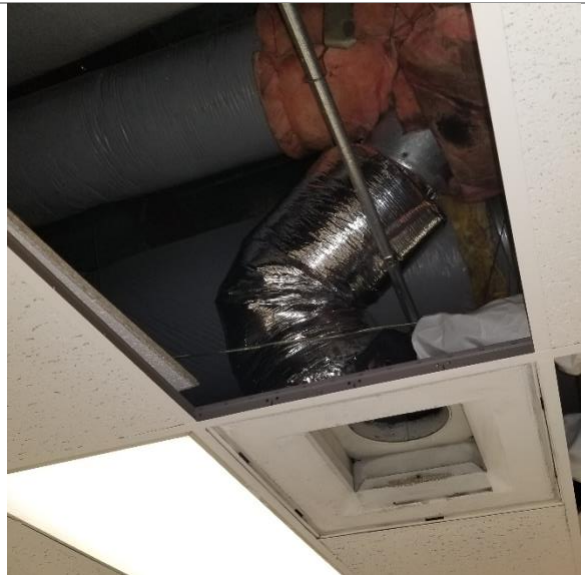
Flex duct replaced (new duct put in)
