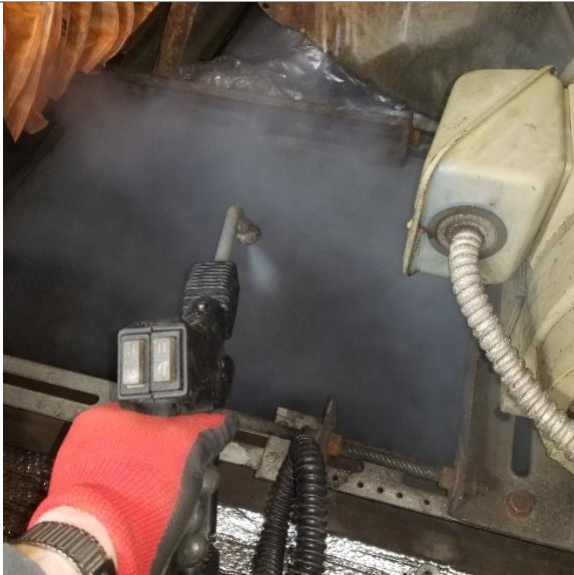
Unit scrubbed and steamed cleaned. Process also eliminates organic growth
