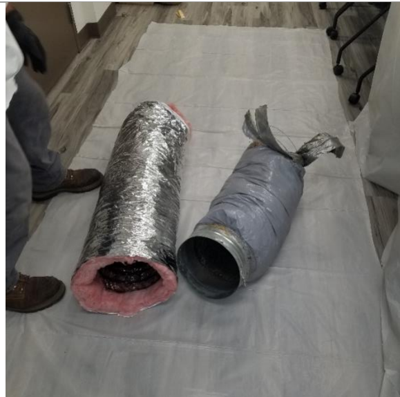
Flex duct replacement (old duct and new duct), meeting room
