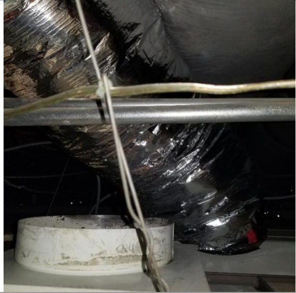
Flex duct replaced (new duct put in)
