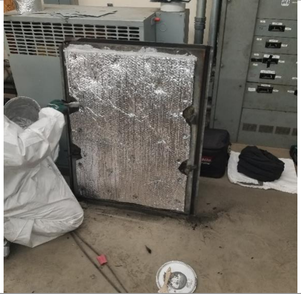
---After--- AstroShield repair to resolve debris issue from doors
