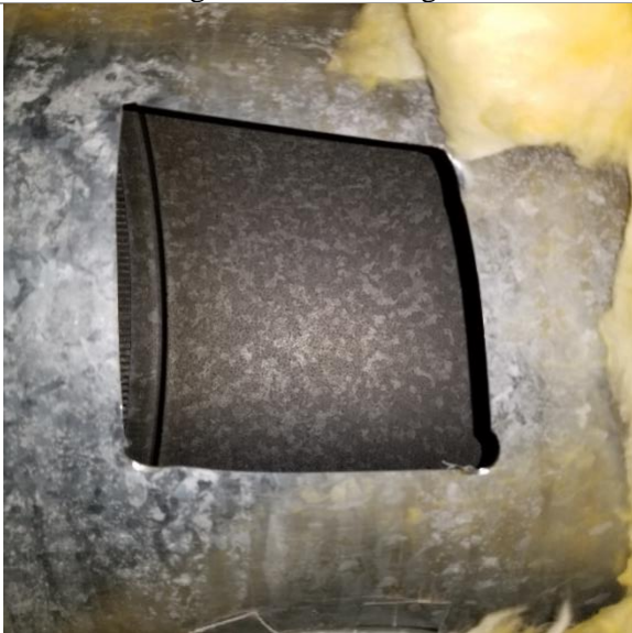
--Before-- Access to main ducts (Typical for all access points)
