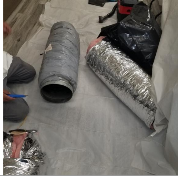
Flex duct replacement (old duct and new duct)
