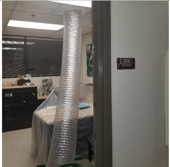
-Methodology- cleaning ducts, HEPA negative air
