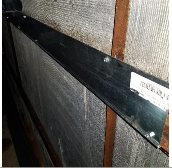
After Complete Metal Addition with Silicon on Edges and Bolted/Screwed Down
