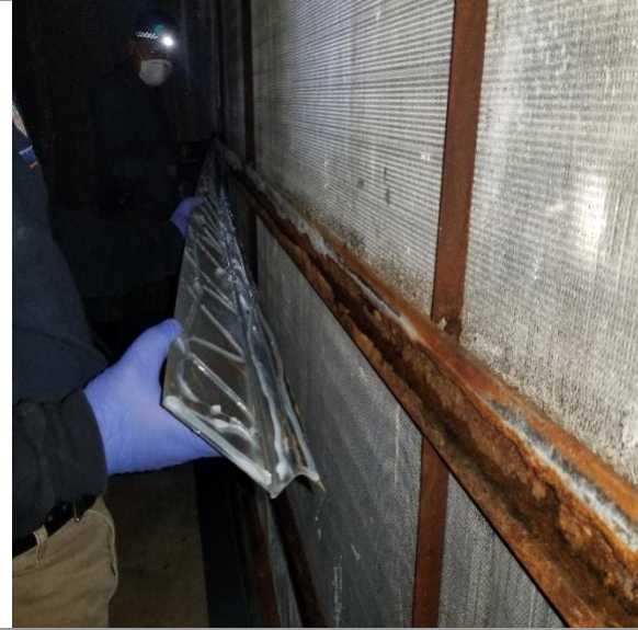
Before Repairs in Progress: In-lay of New Metal with Silicon
