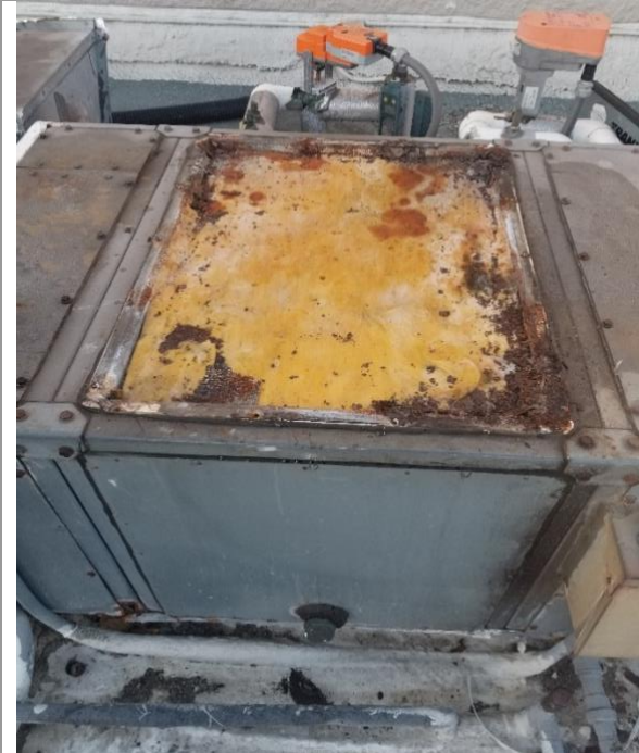
Before Insulation compromised
