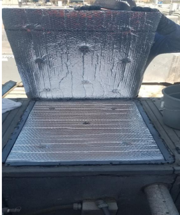
After All insulation replaced with multiple layers of Astro Shield
