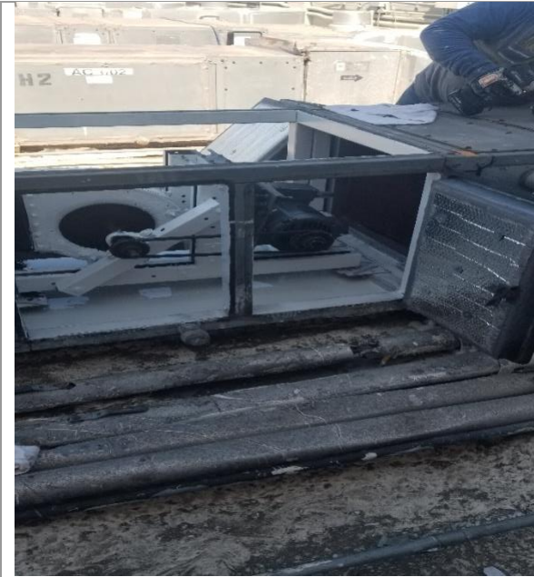
After Fan compartment area with Silver Bullet Epoxy and PC260 (Note all panels with Astro Shield)
