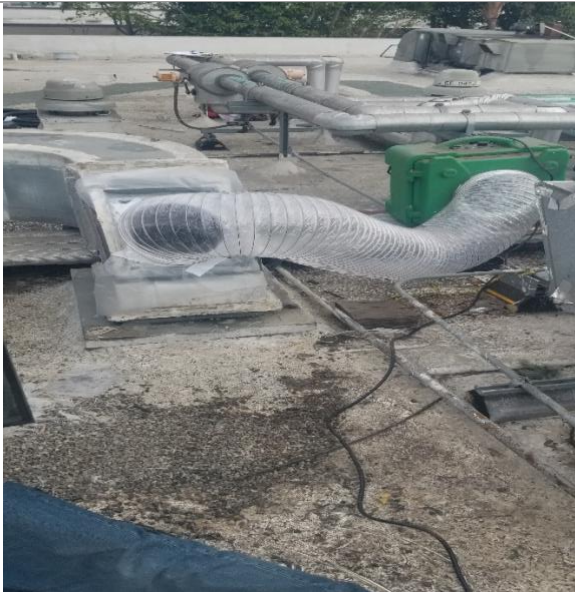
Negative air implemented – Infectious Control
